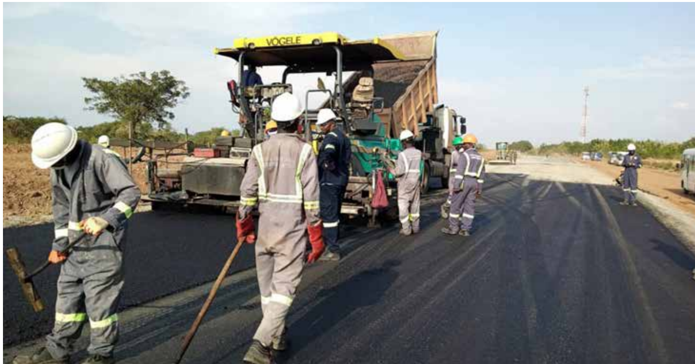
Tilenga Access Roads NETS A1 West Laying Asphalt by Pearl Engineering Company Limited
